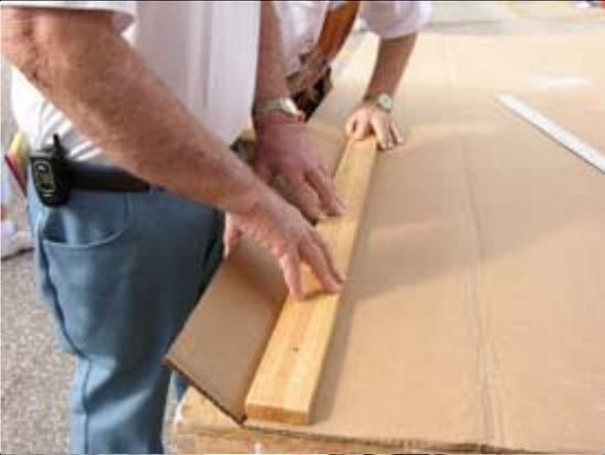
Lay a board along the crushed line and start folding the cardboard a little at a time.
