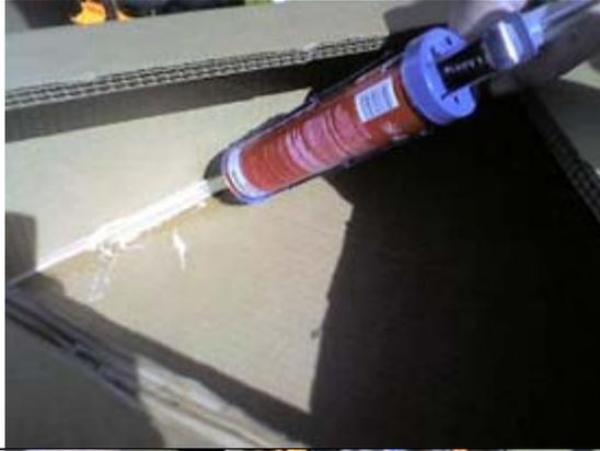
Use construction adhesive to seal all the seams inside the bow and to seal the outside where you cut off the bottom.
