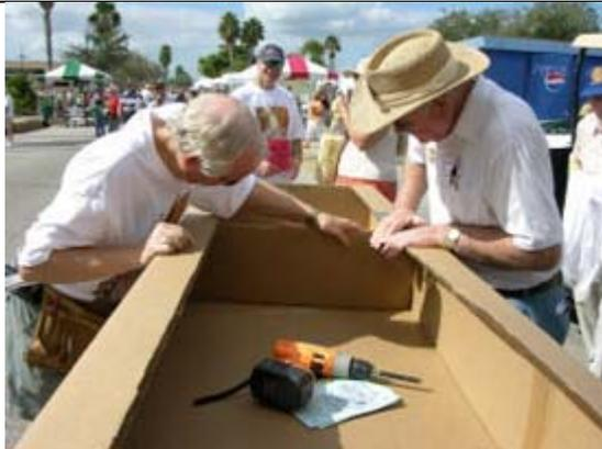
Once the contact cement has dried to where it will not stick to your finger, carefully install the bulkheads. Start by placing the bulkhead on the bottom, followed by the sides and then the top.
