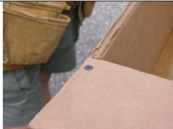
We have found the easiest way to temporarily hold the bulkheads in place is to insert wallboard screws through the outside walls into the bulkheads.
