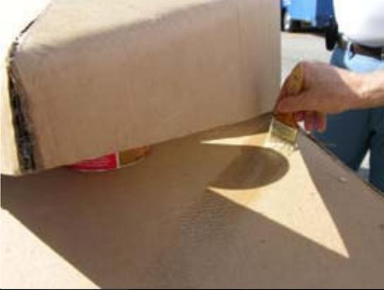
Apply contact cement to the bottom of the boat where it will meet the bow pieces and apply it to the bottom edge of the bow pieces.
