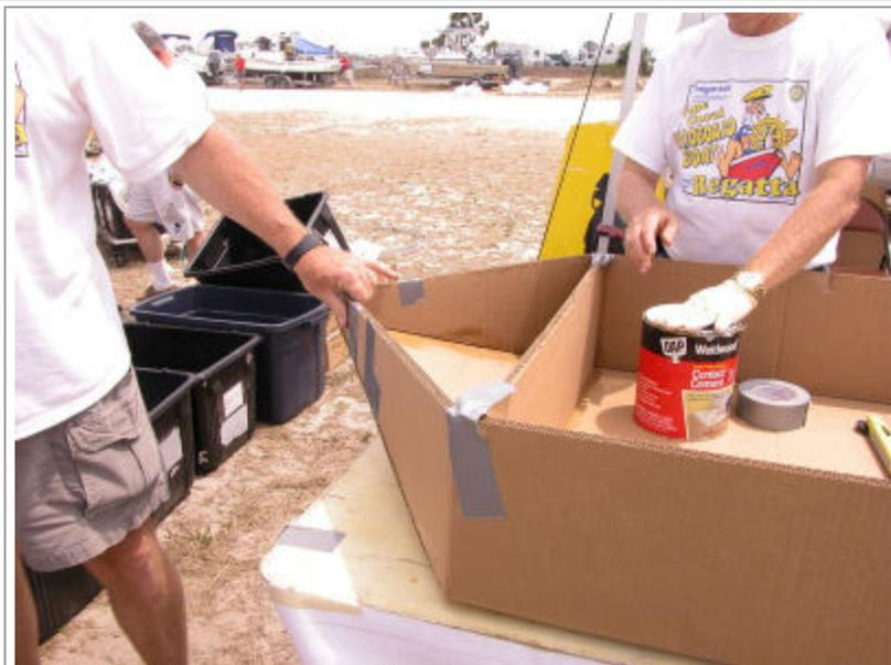
Once the contact cement is dry to the touch, first install the bulkhead and then join the bow pieces together. You can use duct tape to hold the pieces together.
